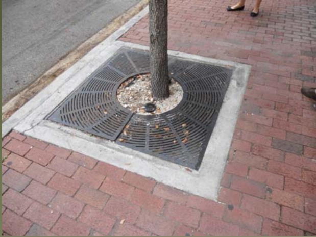
Tree grates with concrete collars and concrete planters
